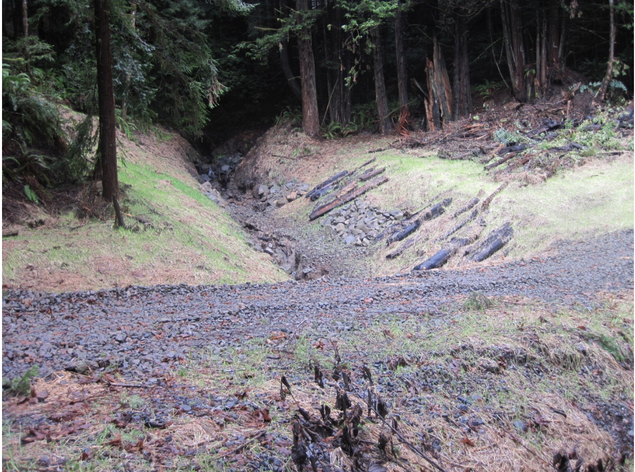
Creek Crossing Upgrade, Road A51.19, Monument Creek Basin, winter BMPEP inspection
